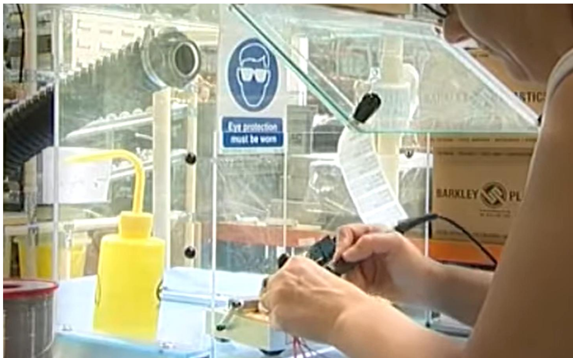
Figure 3: Local Exhaust Ventilation system for a soldering station
